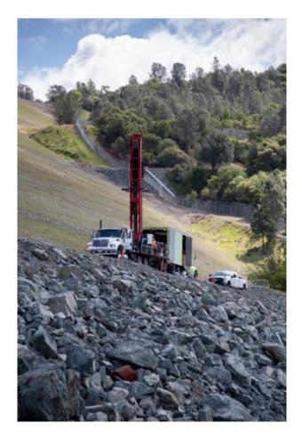
planned piezometer locations include the flood control outlet, the dam toe, the core block and the grout gallery.
