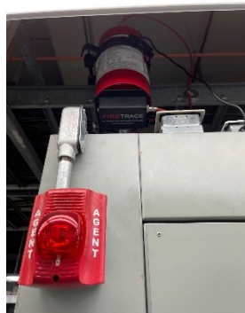
In-Cabinet suppression to protect critical electronics
