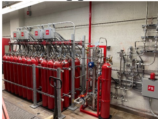
High Pressure Water Mist systems to protect oil processing areas
