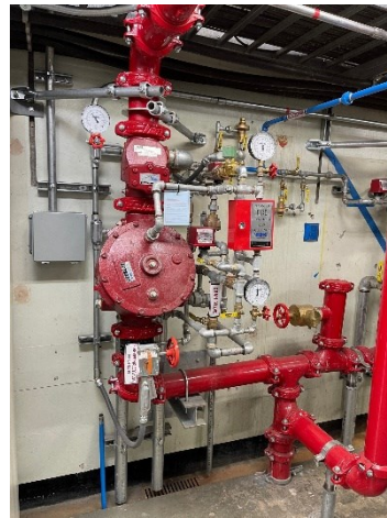
Pre-Action riser system to control activation of water based sprinkler systems
