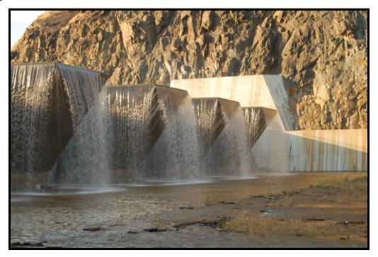
Spillway Fuse Gates at Terminus Dam
