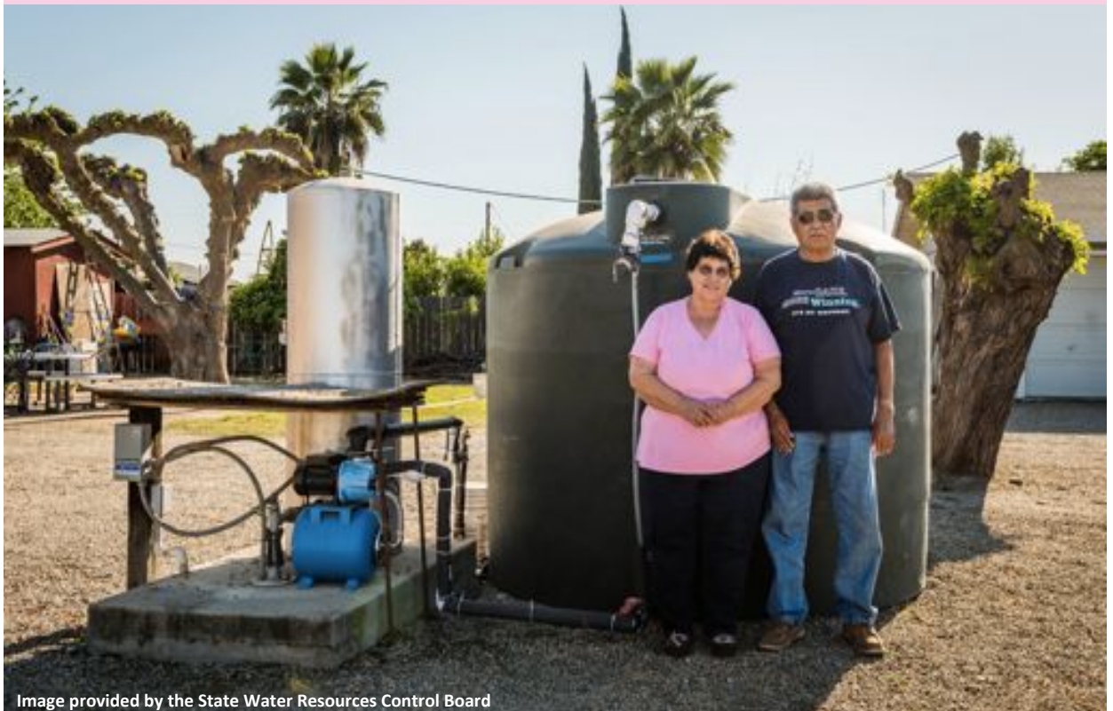
Image provided by the State Water Resources Control Board
