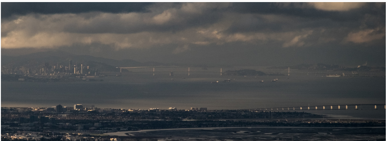
Figure 8.4 When the State borrows to pay for infrastructure, roughly one out of every two dollars spent on infrastructure investments pays interest costs, rather than construction costs. (Photo: three bridges; Justin Dolske, flickr, licensed under Creative Commons license 2.0)
