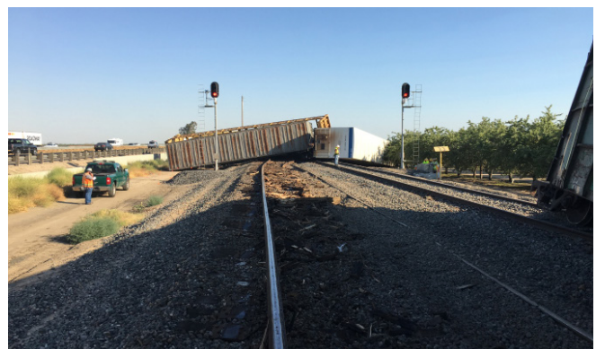
Figure 3.7 Extreme heat can cause buckling of railroad tracks and lead – as in this example from Tulare County in June 2017 – to derailment. (Source: California Department of Fish and Wildlife, used with permission)
