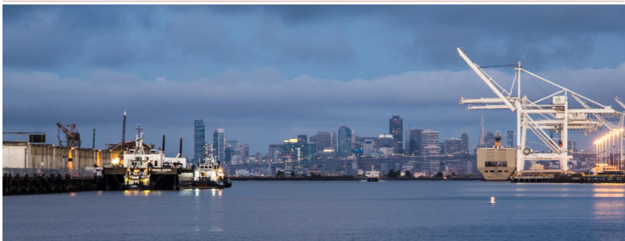
Figure 3.13 Ports, airports and telecommunications infrastructure – while not State-owned – are critically important to the state’s functioning and economy. Many of these infrastructure systems are increasingly at risk from flooding, sea-level rise, wildfires and other extreme events. (Photo: San Francisco skyline and Port of Oakland, Tony Webster, flickr , licensed under Creative Commons license 2.0)
