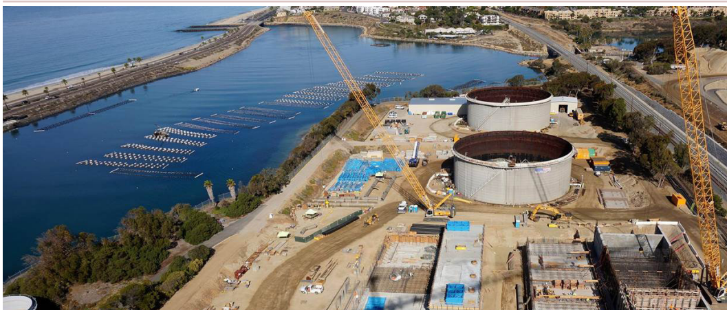
Figure 10.6: Many infrastructure decisions involve difficult trade-offs and engineers and architects need to have the skills to effectively convene, facilitate and navigate stakeholder conversations. (Photo: Carlsbad, California, desalination plant; vanderhe1, flickr , licensed under Creative Commons license 2.0)
