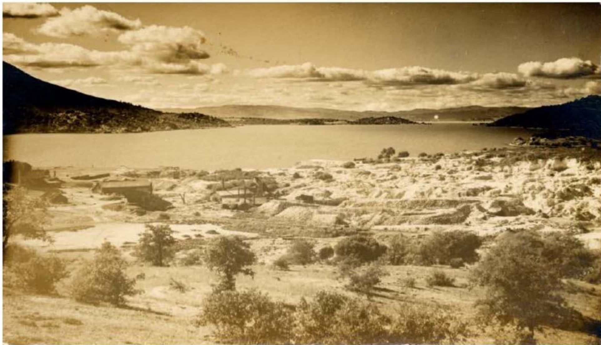
PLATE 2. Mercury-laden mine tailings and waste rock piles at the Sulphur Bank Mercury Mine ca. 1900, before more modern earthmoving equipment and bulldozing occurred (courtesy of Lakeport Historic Courthouse Museum).
