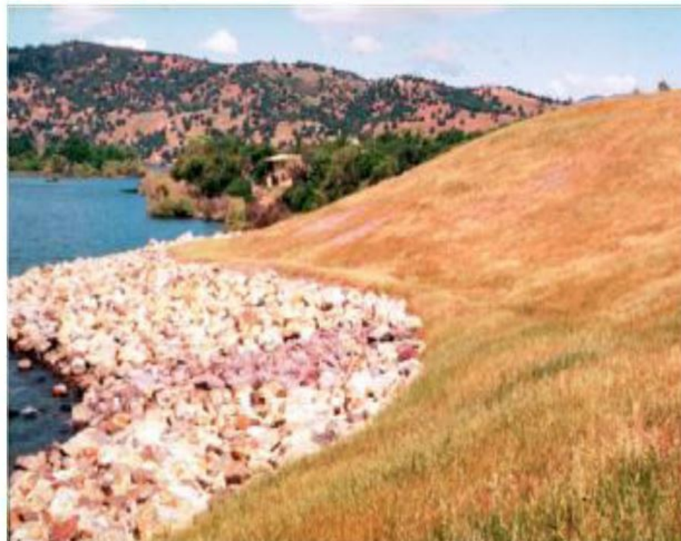
PLATE 9. Waste rock piles from the Sulphur Bank Mercury Mine along the Clear Lake shoreline. (Left) Before the 1992 U.S. EPA shoreline remediation. Note the steeply sloped waste rock pile that eroded mercury-laden soils into Clear Lake during heavy rains. (Right) After the 1992 remediation. Note the vegetated slope, reduced angle of the piles and rip rap along the shoreline to reduce erosion.
