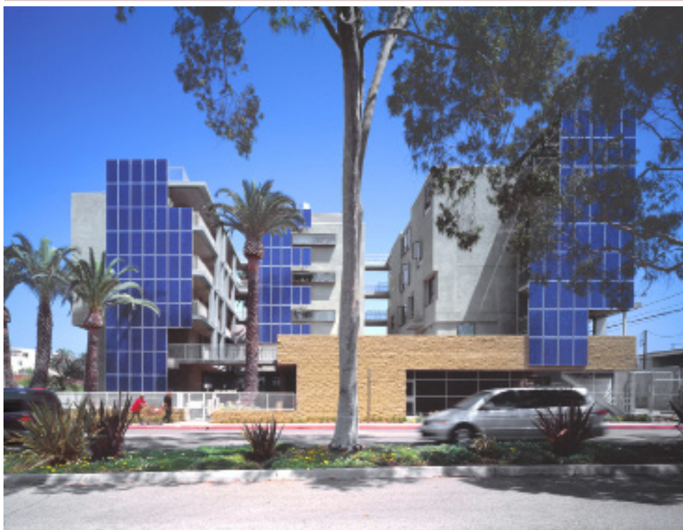
Figure 7.8: Integrated infrastructure development can create many synergies and co-benefits. This multi-family housing unit, known as Colorado Court, in Santa Monica was the first LEED “Gold” certified multi-family building in the U.S. It combines many sustainability features and provides affordable housing to lower-income residents. (Photo: Calder Oliver, Wikimedia Commons , licensed under Creative Commons license 2.0)
