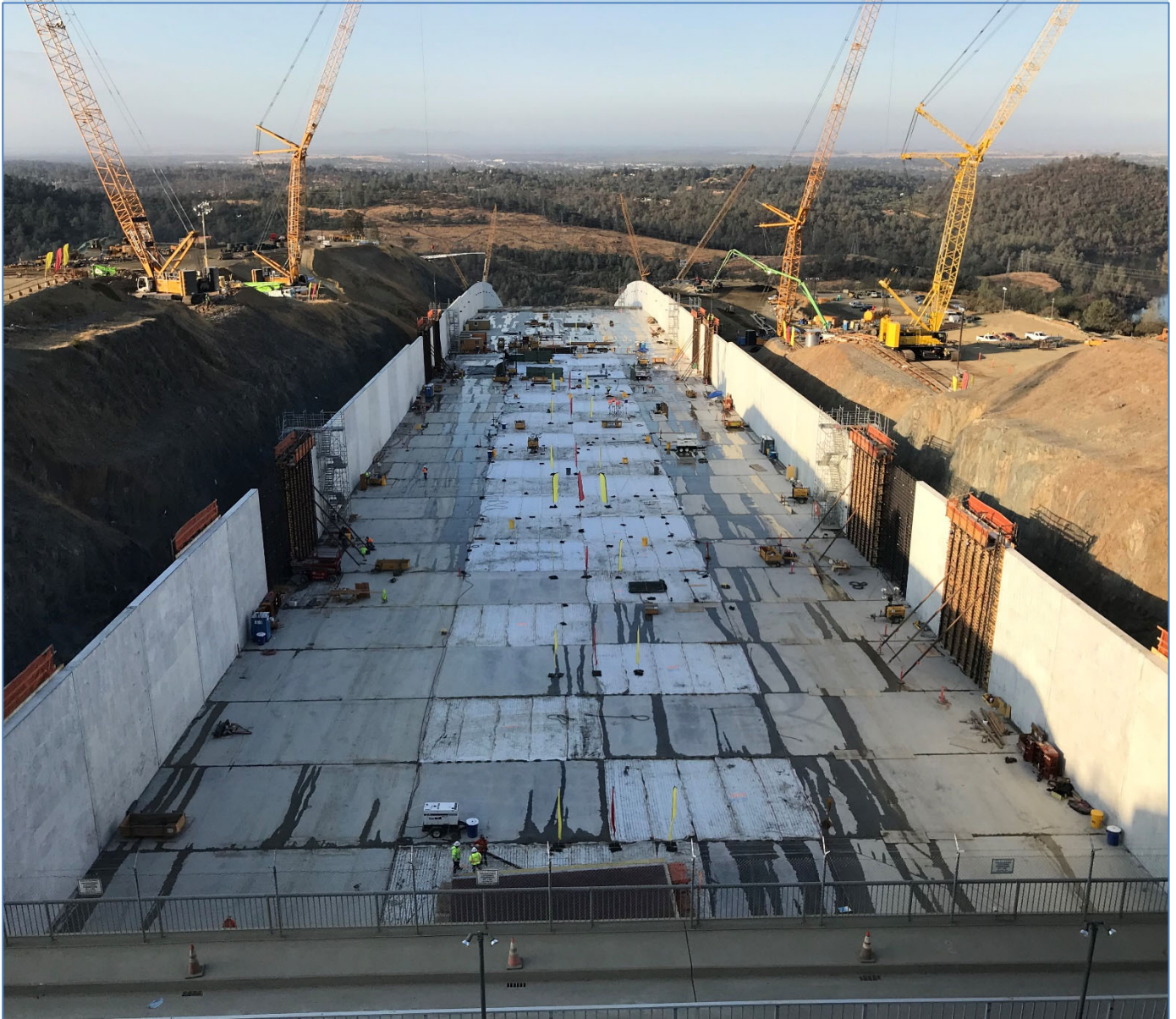
Figure 1. Construction of chute slabs and walls in the upper section of FCO chute.
