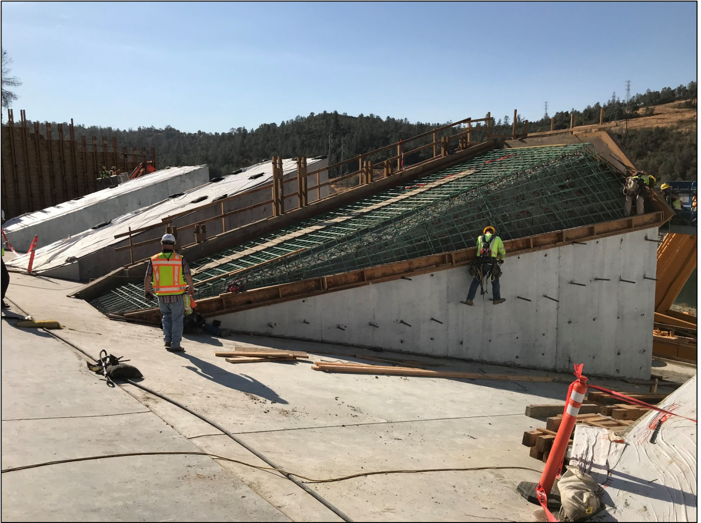
Figure 5. Reconstruction of the dentates at downstream end of FCO chute.
