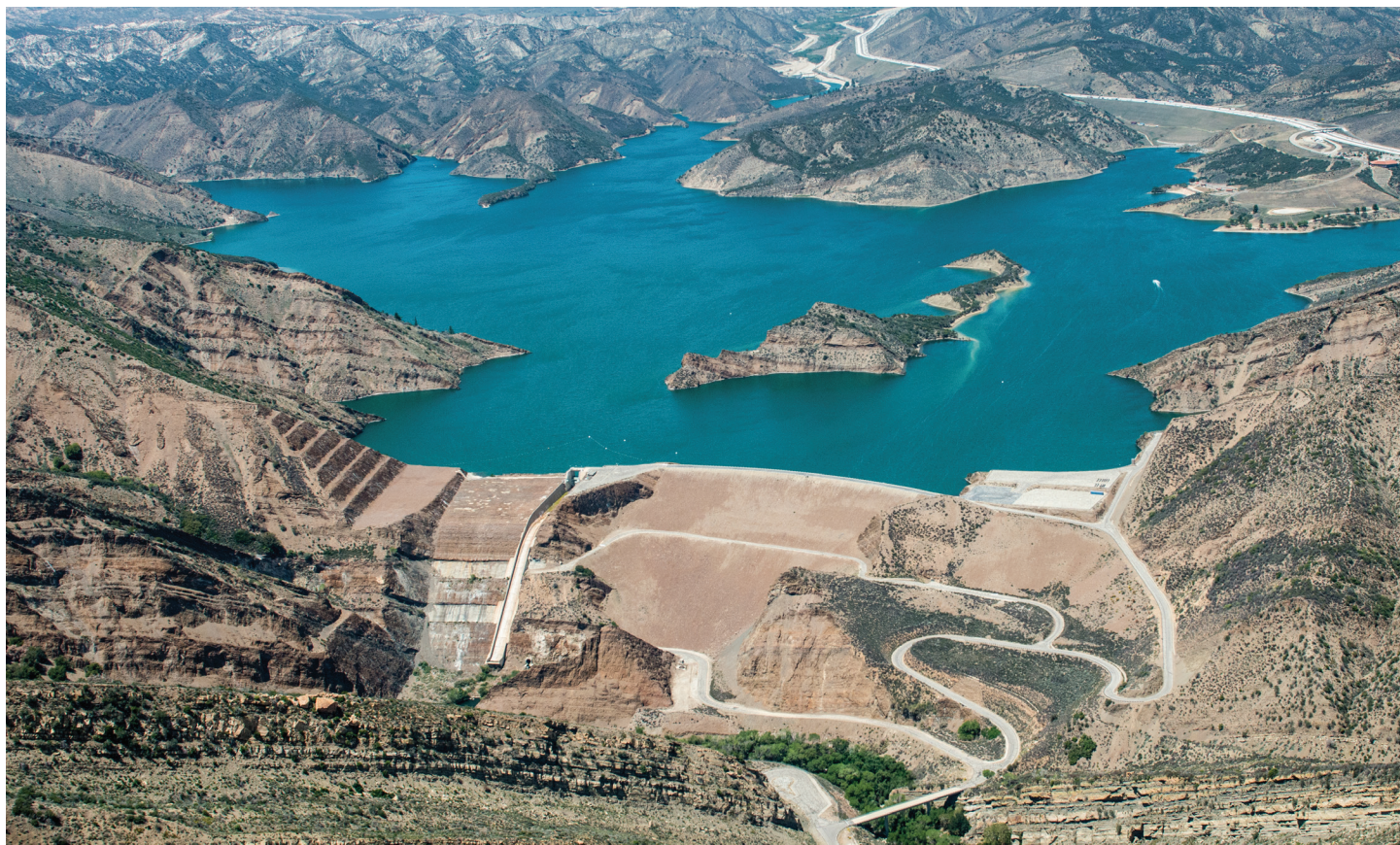
This aerial view looks north toward Pyramid Dam and Pyramid Lake located on Piru Creek in Los Angeles County. Source: Florence Low – California Department of Water Resources
