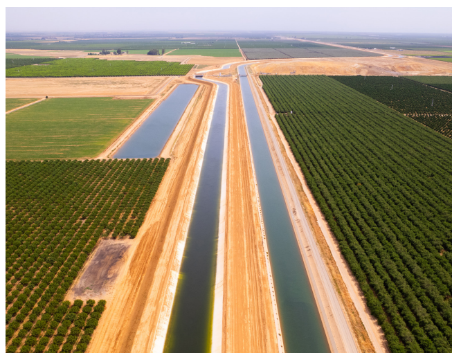
Figure 3. Newly constructed canal next to original Friant-Kern canal after subsidence reduced original capacity by 60% in some areas of the project.
