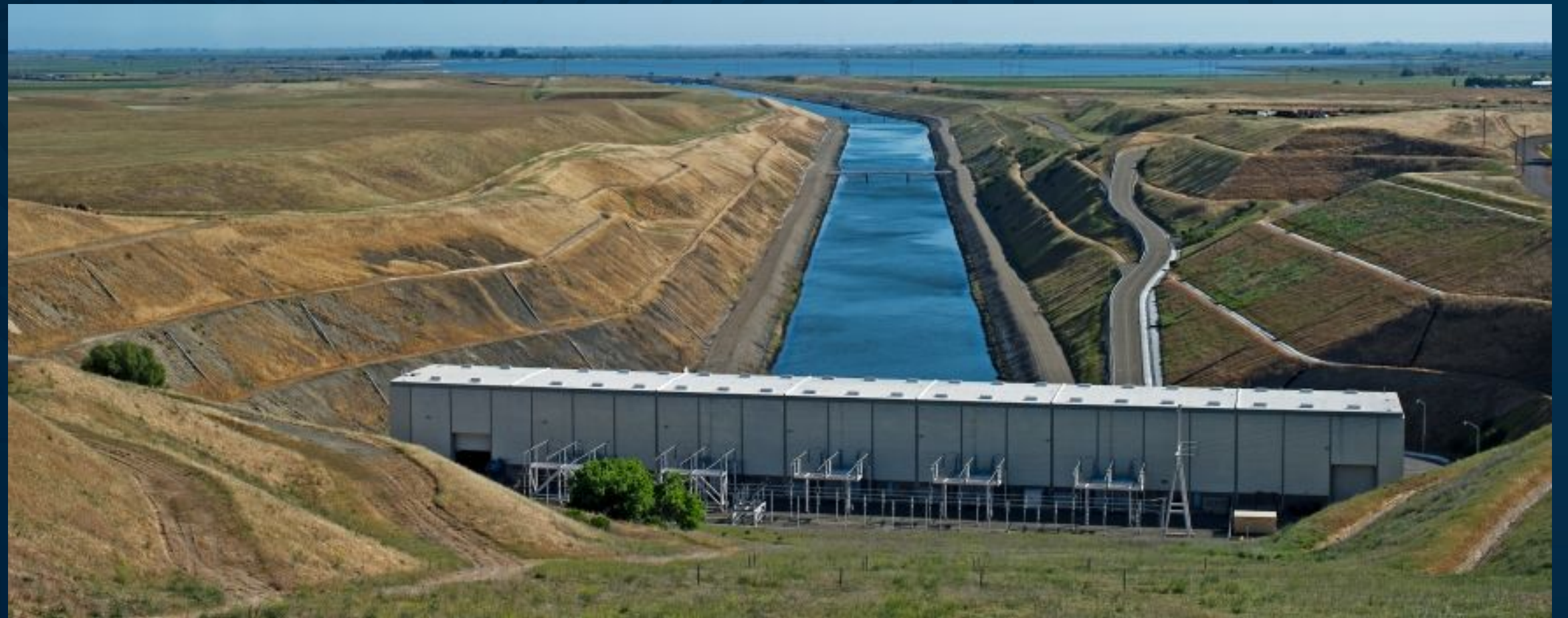
Harvey O. Banks Pumping Plant
