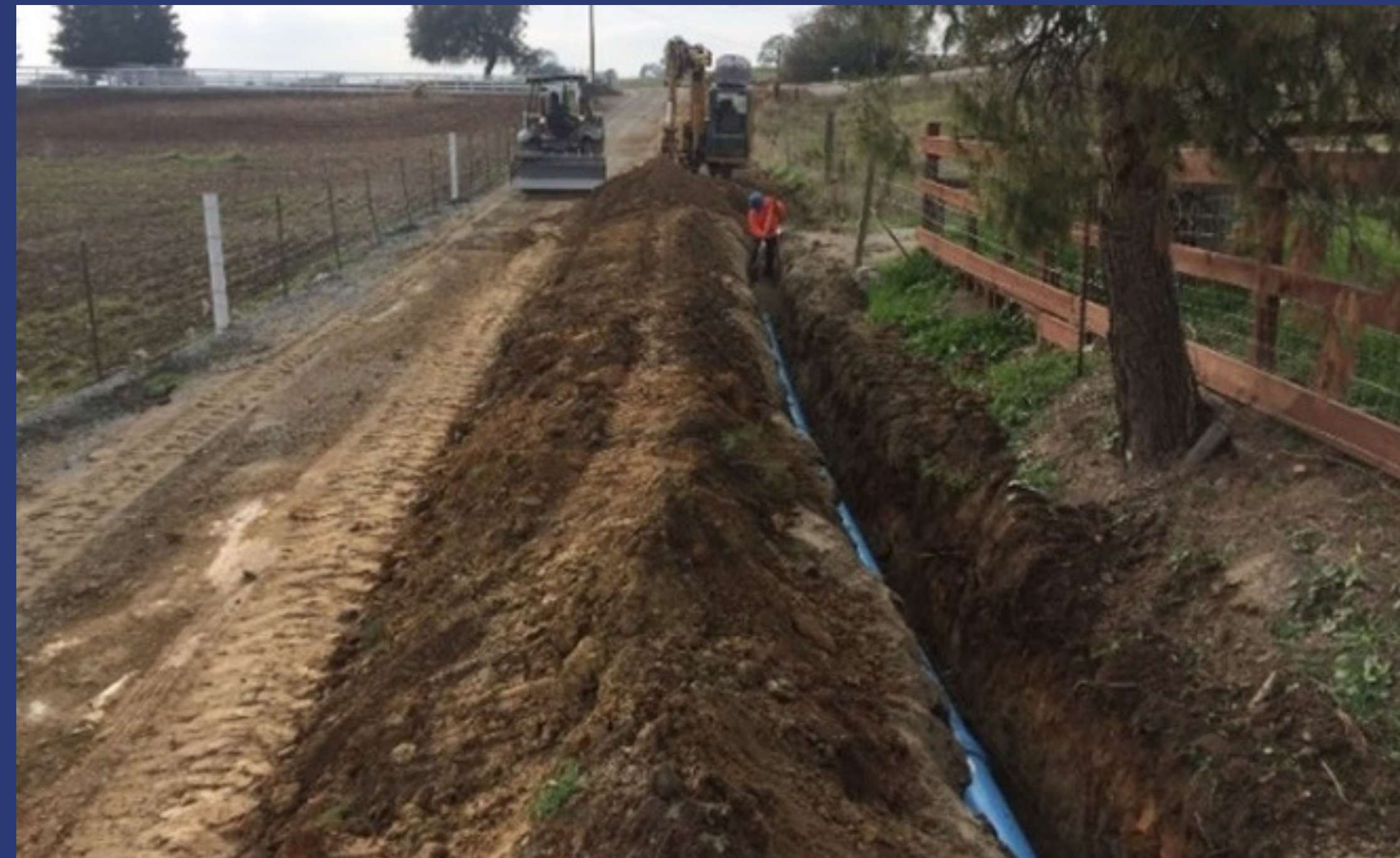
Quartz/Stent water main extension - 2016
