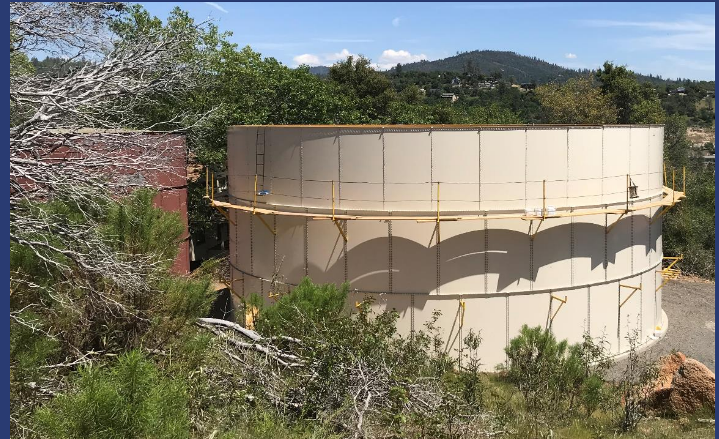
New Mono Vista Water Storage Tank, June 2020 (One step closer to water storage tank consolidation)
