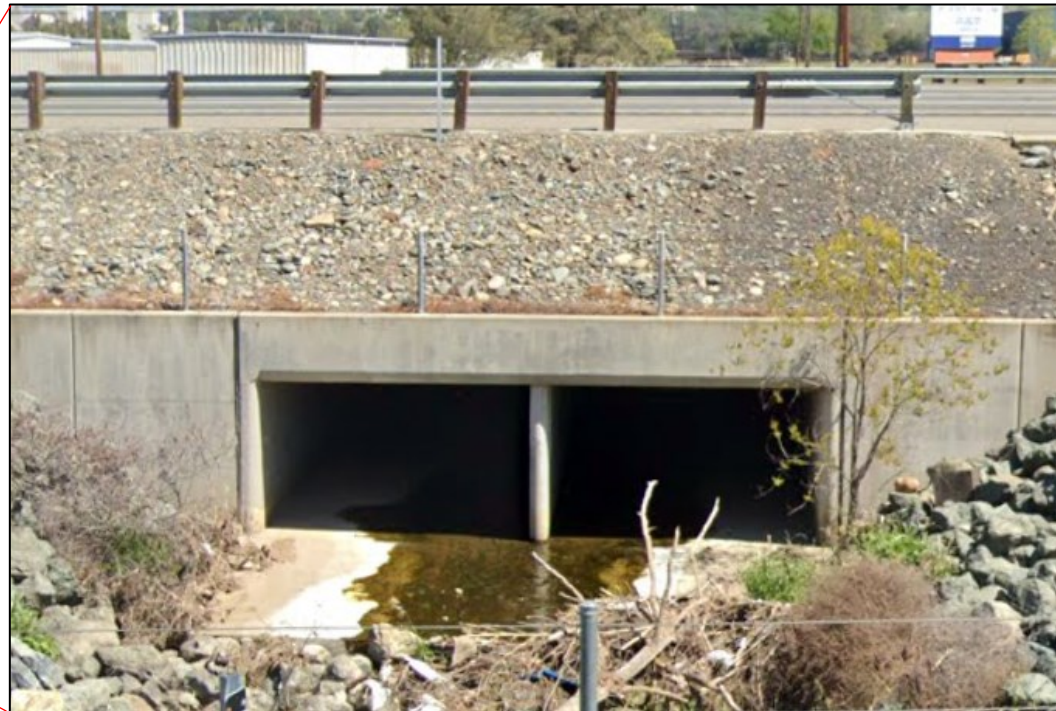
Twin box culverts along dry Creek beneath Hwy 70
