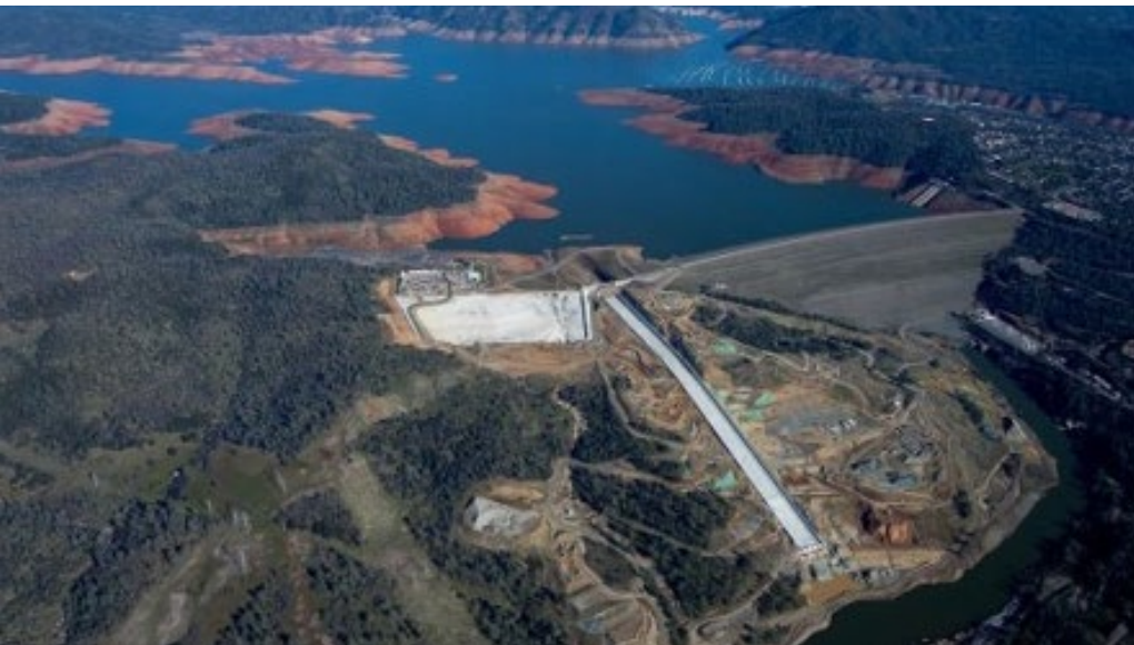
Aerial view of the Oroville Dam main spillway. During an active water release, high-velocity water flows through the concrete-lined chute into the diversion pool below.
