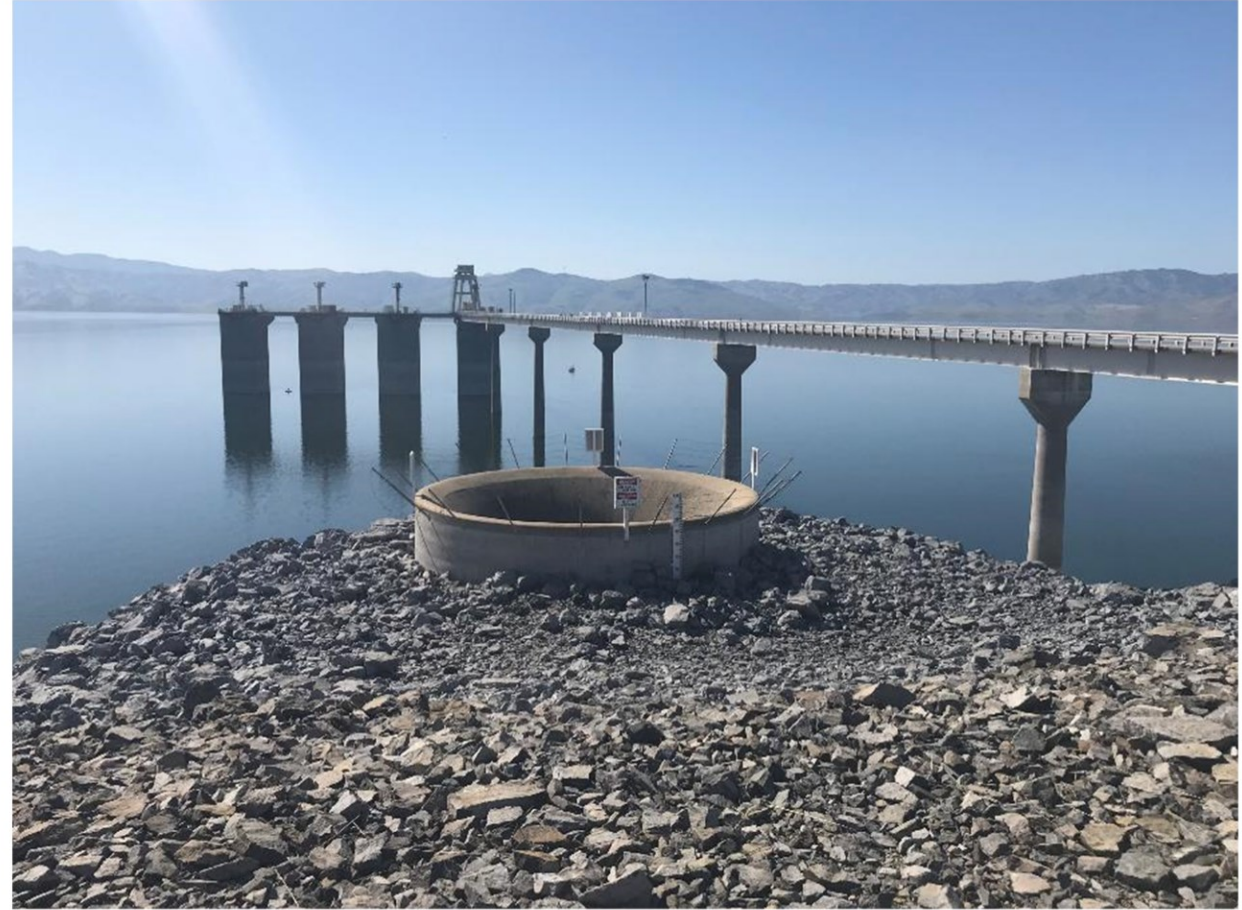
B. F. Sisk Dam (San Luis Reservoir) Glory Hole Spillway and Gianelli Pumping-Generating Plant Intake Structure
