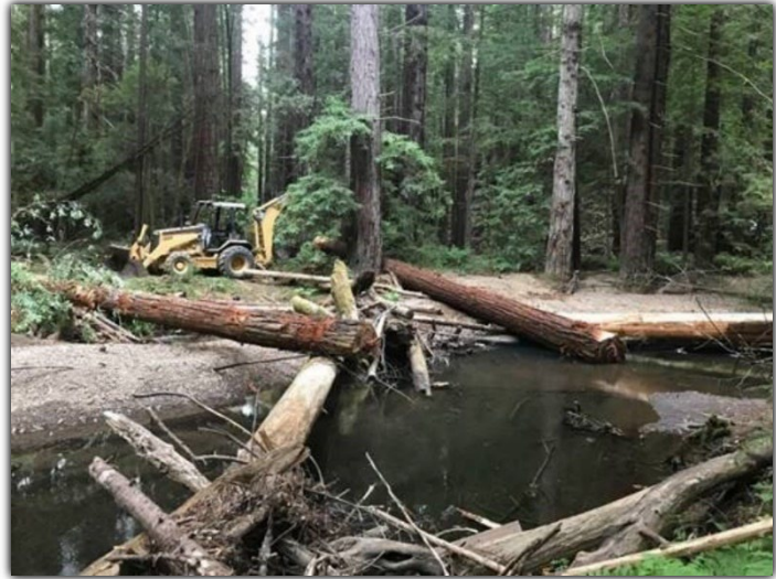
Image 2: Restoration of salmonid habitat conditions and water quality through large wood augmentation in critical Coho salmon and steelhead streams and rivers (Mendocino Coast Large Wood Augmentation Project Phase 1, Trout Unlimited)
