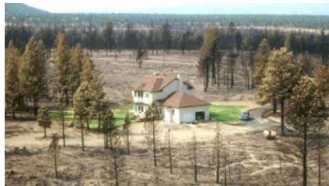
Figure 3: Home surrounded by wildland that survived a fire due to good defensible space.
