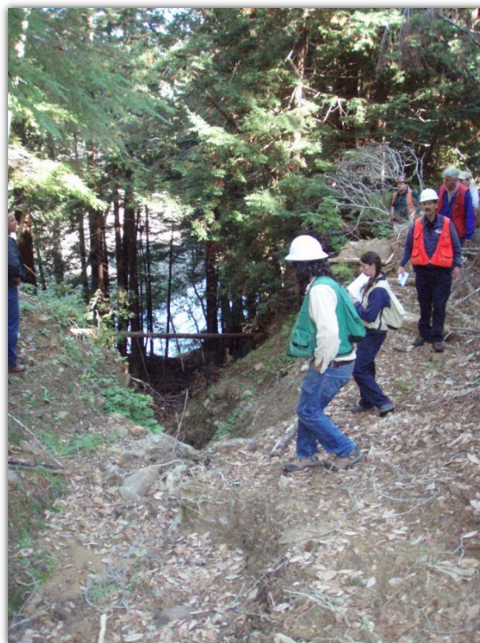
Image 1: Review team inspecting drainage and erosions issues proximate to harvest site.
