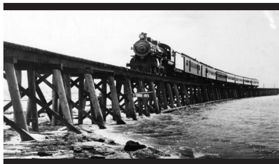
During the 1905-1906 Colorado River Flood, a southern Pacific passenger train crosses the Salton Sea on a trestle at a point 5 miles east of Salton Station. Bureau of Reclamation photo 1905.
