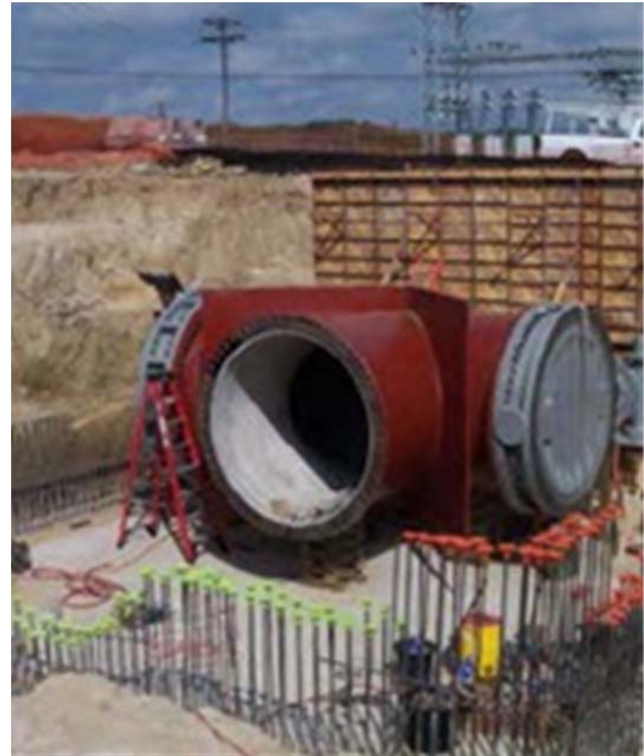
AECOM completed the fast-track repair and replacement of the Lake Tawakoni 84-inch-diameter main on time and within budget.
