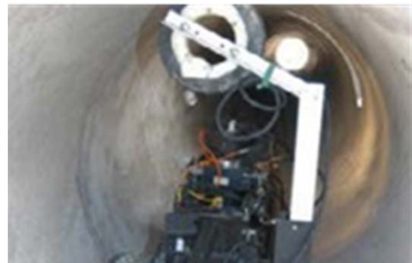
The EM technology allowed DWU to confirm, on site, that the correct pipe segments had been located. This turnaround was critical to help minimize pipeline shutdowns.
