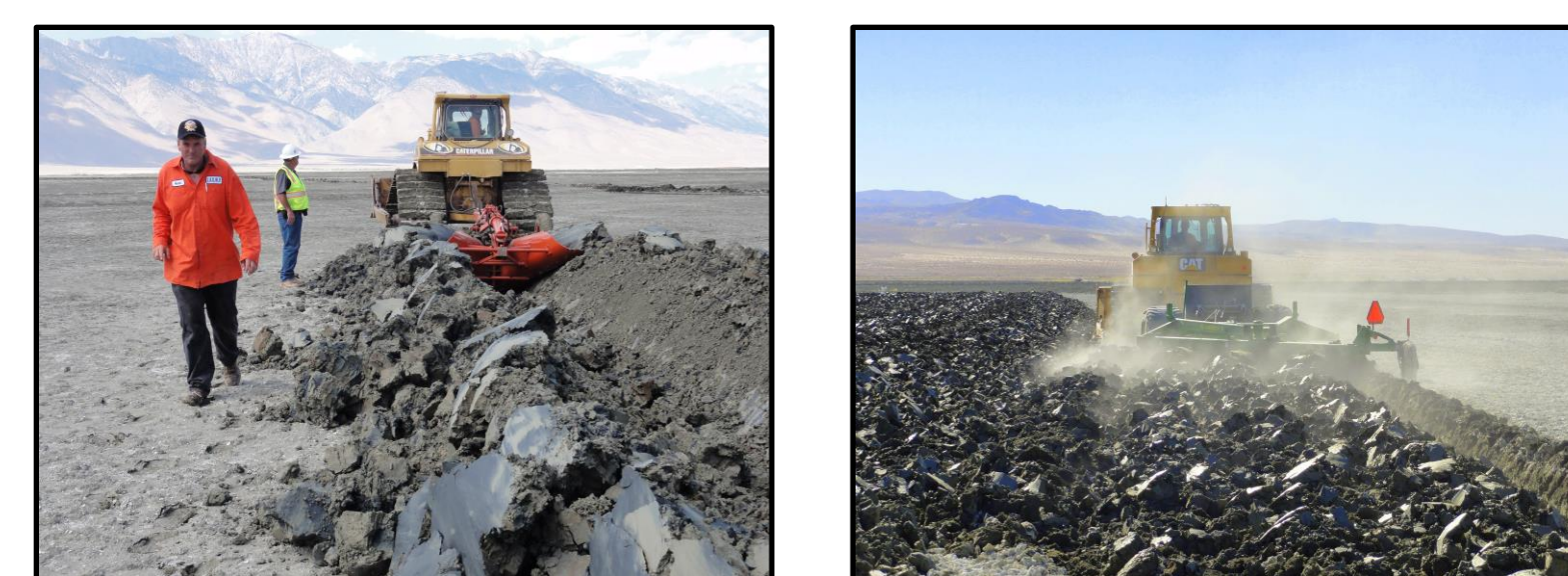
Figure 3. Photograph of a Bull Plow (left) and Switch Plow
