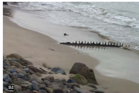
Deteriorated Steel Groin Hazards Las Tunas County Beach, Malibu, Los Angeles County
