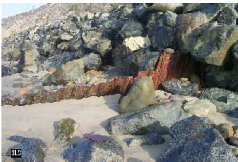
Deteriorated Steel Groin Hazards Las Tunas County Beach, Malibu, Los Angeles County
