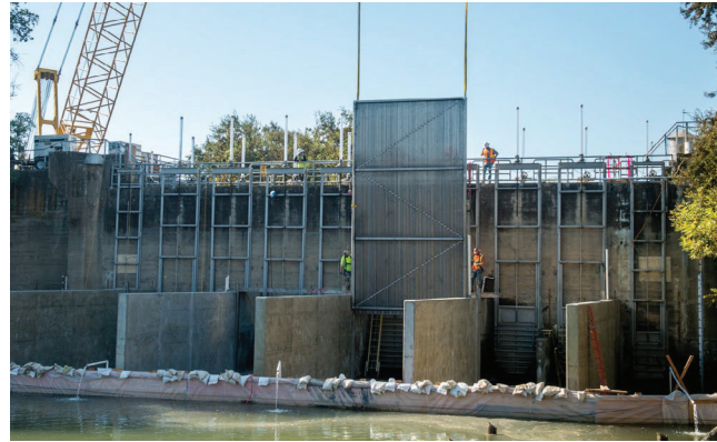
Part of California EcoRestore, the Knights Landing Outfall Gates Fish Barrier Project prevents salmon from entering Colusa drainage canal so they can continue migrating in the Sacramento River.
