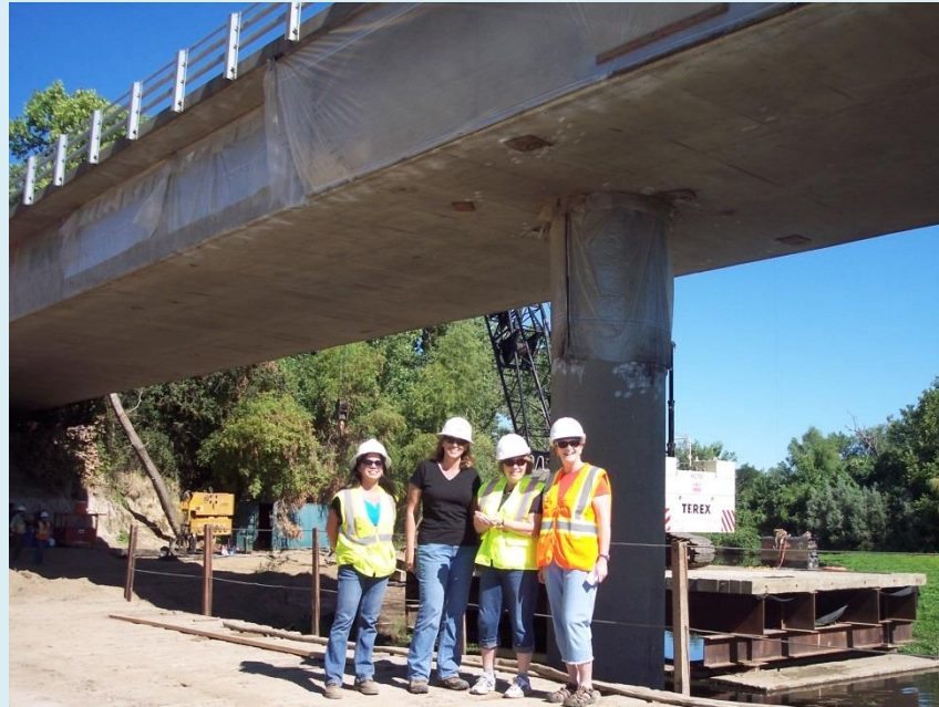
Ord Ferry Bridge Bat Colony Restoration Project
