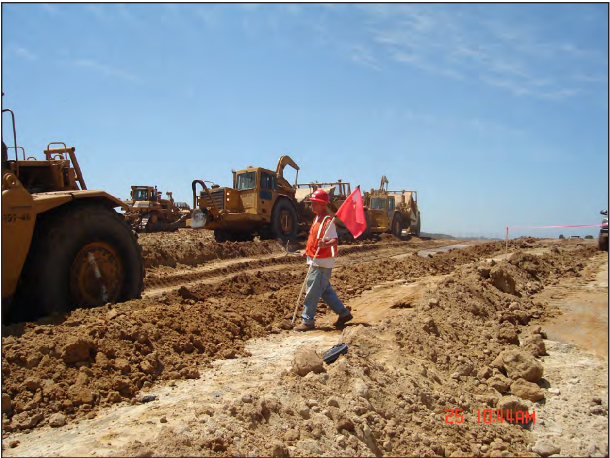
FIGURE 3. Field paleontologist Pat Sena monitoring mass grading activities in upper Pliocene strata of the San Diego Formation as exposed during construction of residential housing in coastal San Diego County. San Diego Natural History Museum, Department of PaleoServices photograph.
